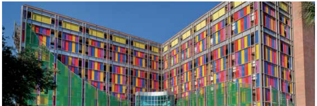
Small wire mesh elements clad the old brick structure. Shands Children's Hospital, Gainesville, USA.
