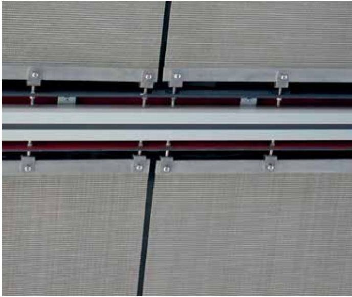
Fixed mounting system for ceiling with flat tension profiles and clevis screws.
