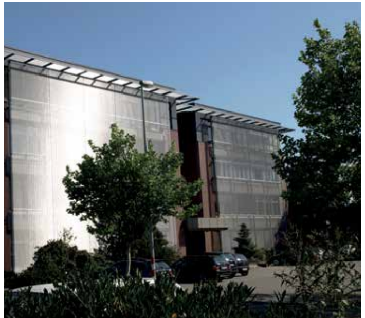
DOGLA-TRIO blends the newly-added floor with the existing structure. Haver & Boecker, Oelde, Germany.
