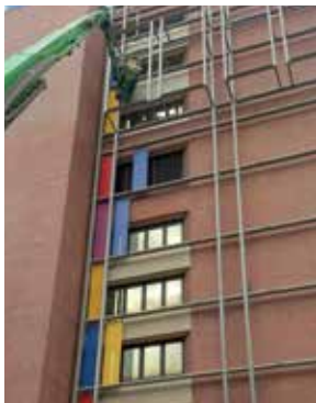
Small wire mesh elements clad the old brick structure. Shands Children's Hospital, Gainesville, USA.
