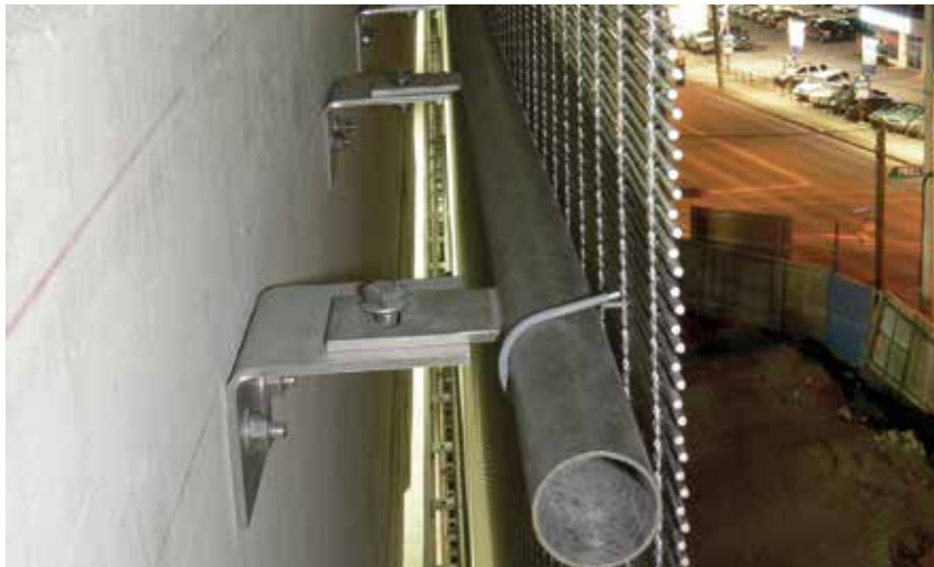
Intermediate mounting: Round tube and wire connectors.
