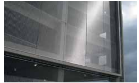
Owing to its transparency, stainless steel mesh allows natural circulation of air.
