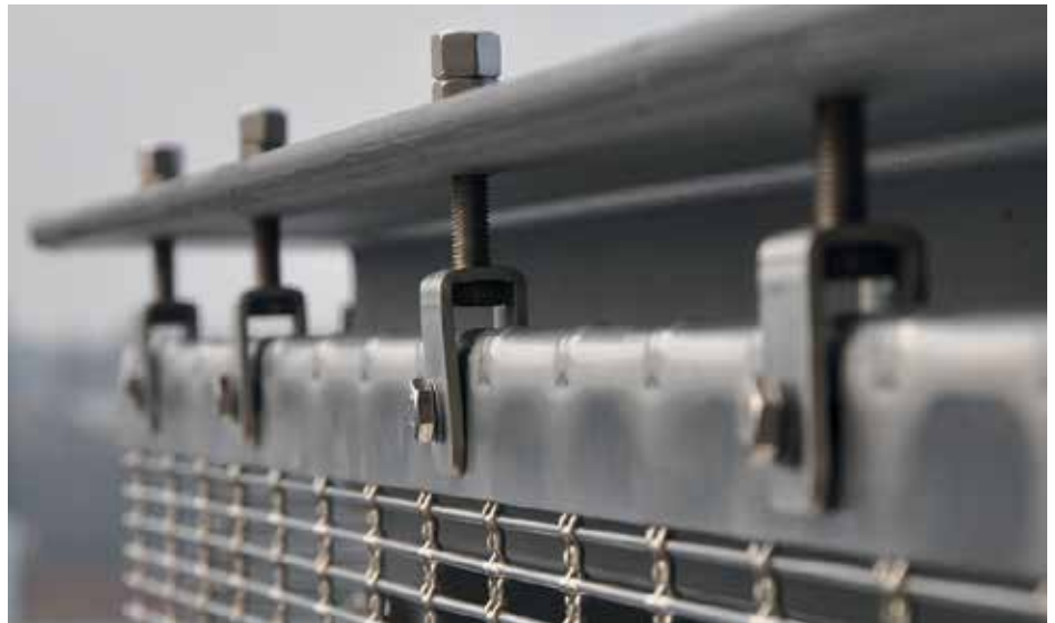
Top mounting: Flat tension profile and clevis screws.
