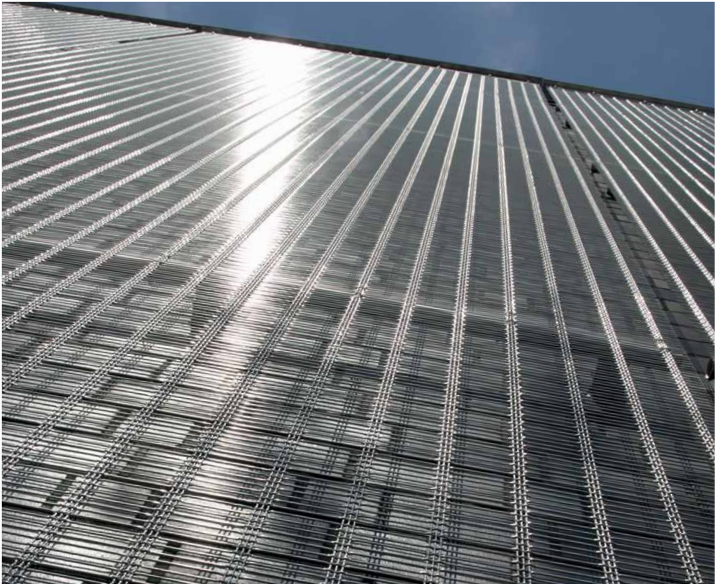
Architectural mesh tensioned over several stories. Load-bearing substructures are only required on the upper and lower face.
