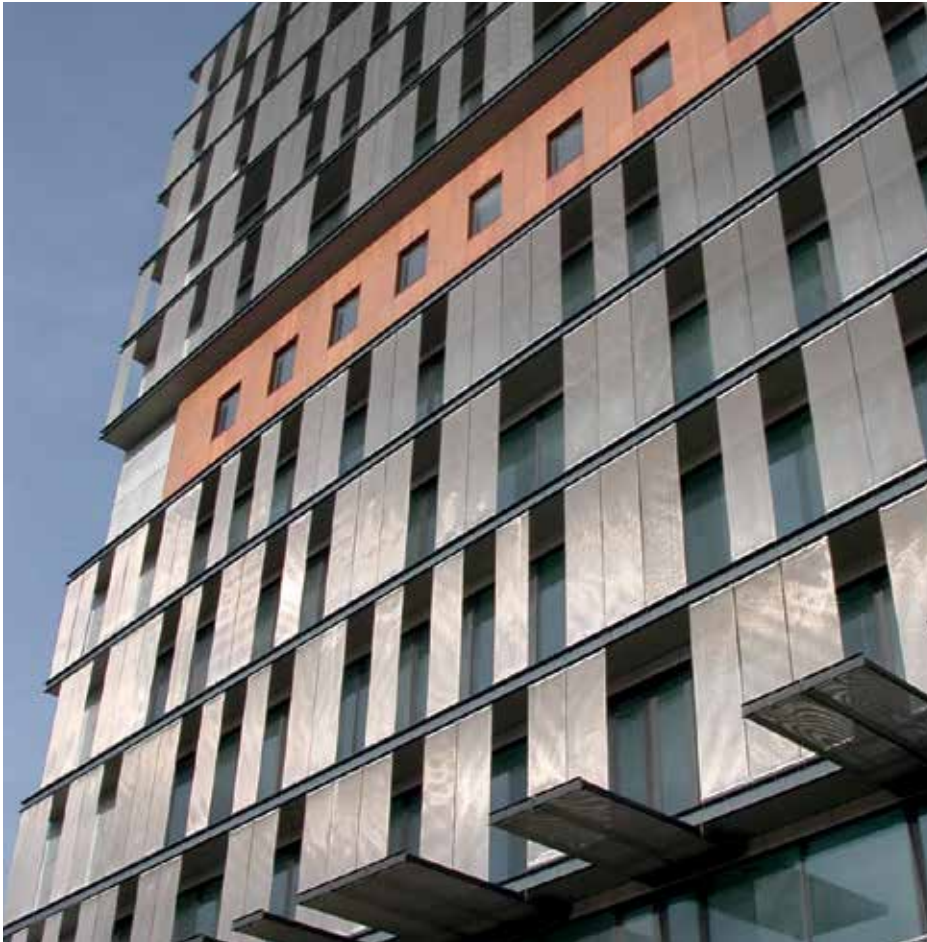
Transparent architectural mesh elements effectively blends sun protection with limitless design possibilities
