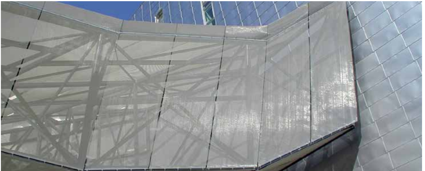
Three-dimensional canopy with individually-tensioned elements. Malaga Exhibition Center, Spain.
