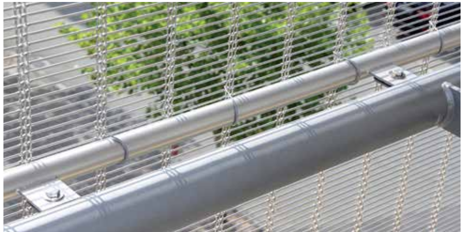
Intermediate mounting: Round tube and wire connectors.
