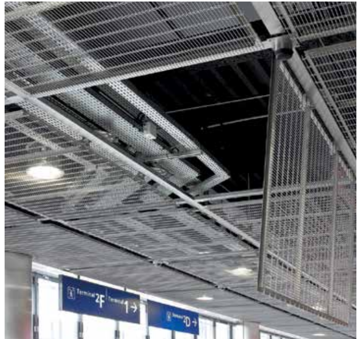
Removable mounting system for ceilings without sag and with framed elements.
