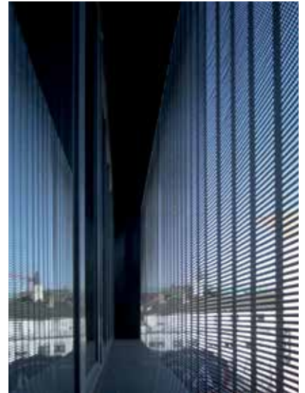
The open geometry of the architectural wire mesh preserves the view of the outside world.
