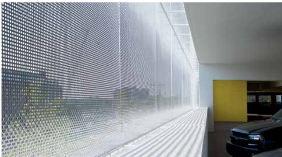
Sun protection combined with an unobstructed view from inside. Car park, Chesapeake, USA.
