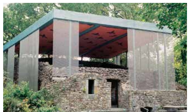
A semi-transparent stainless steel mesh encloses the existing building and ensures natural lighting. C&A Eco Store, Mainz, Germany.
