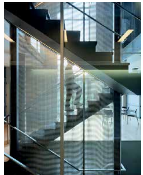
Stairwell cladding using two layers of architectural mesh to create moiré effect. McGill University, Montreal, Canada
