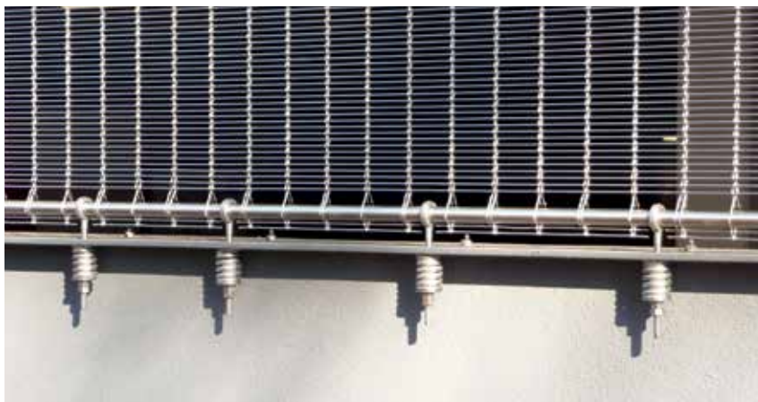
Bottom mounting: Round bar with eyebolts and pressure springs.
