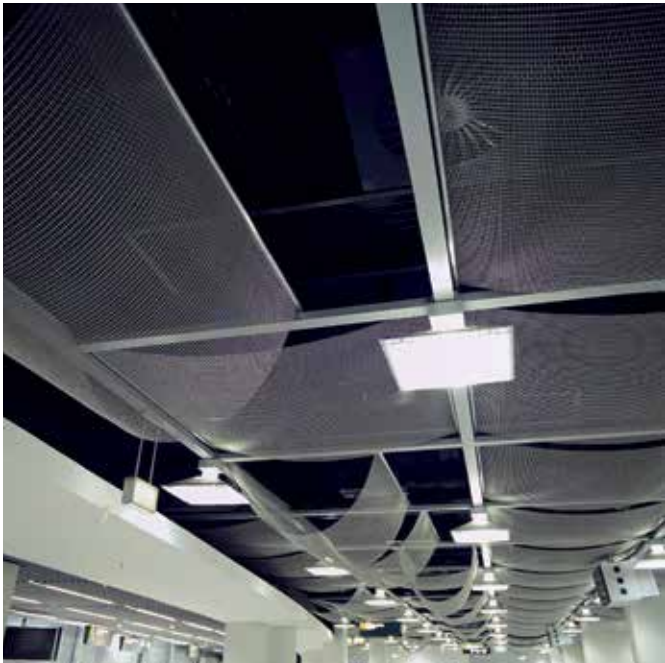
Adjustable mounting system for ceilings with sag.
