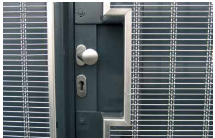
Mesh with edge-protection profiles.
